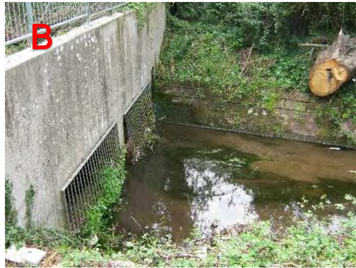
Plate 3.13 - A. North Purbrook Heath looking upstream (east) towards A3 / London Road (467150, 107790); B. Screened culverts where North Purbrook Heath exists culvert under A3/London Road (467180, 107780)
