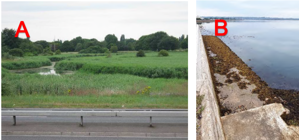
Plate 3.30 - A Looking west across A2030 / Eastern Road towards the onstream ponds of Great Salterns Drain (467650, 101790); B. looking north along the tidal defence adjacent to A2030 / Eastern Road downstream of Great Salterns Drain (467670, 101790)
