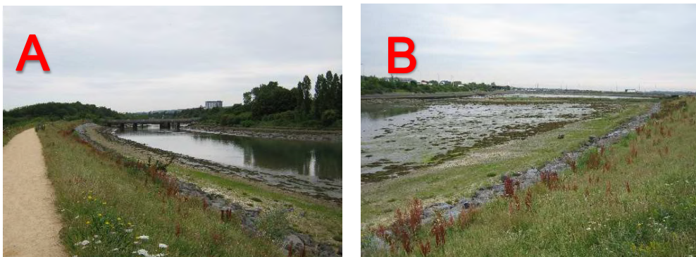
Plate 3.29 - A. Ports Creek looking west (466980, 104090); B. Ports Creek looking east towards A2030 and main body of Langstone Harbour (466980, 104090)
